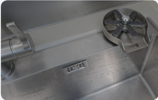
Tumbler Washing Machine Installation
